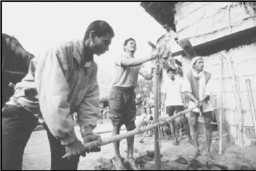
*Sinking a tubewell using the sludging method. The work is led by Bipta Chaudray (centre) who is the skilled labourer.*
