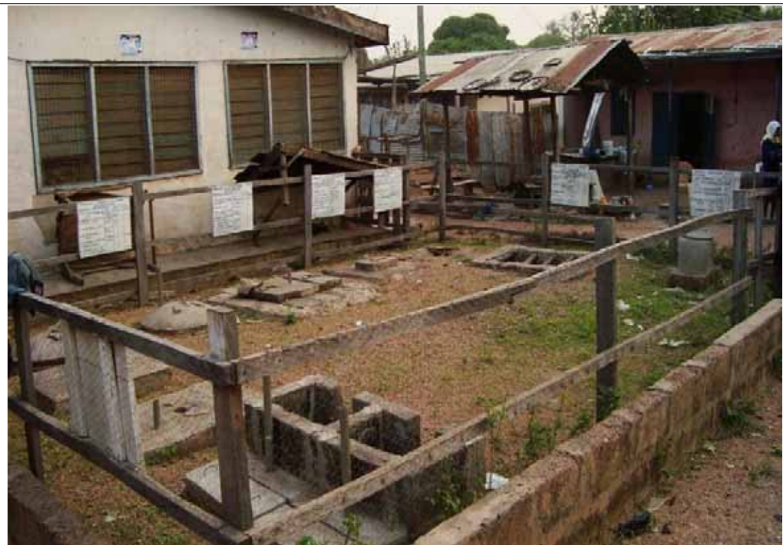
Plate 1: The Krachi Sanitation Information Centre (also served as a sanitation market) from where beneficiaries selected the types of latrines to be constructed for them.
