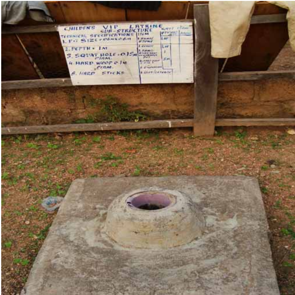
Plate 9: Children VIP Latrine
