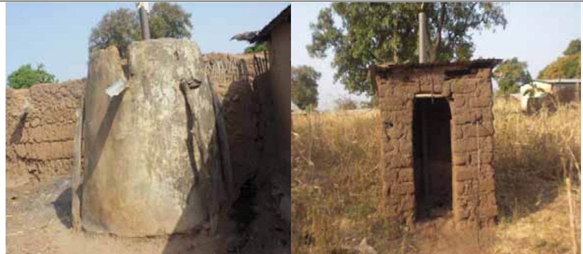
Plate 1: different structures housing the latrines captured during the field work. The structures are mostly not plastered. They also have no doors, thus snakes and scorpions are likely to enter into them especially at night.
