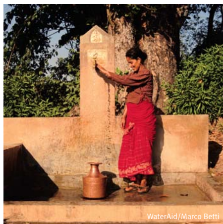
A tapstand supplied by a gravity flow scheme in the mountains of Nepal.
