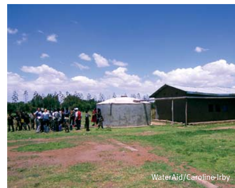
A roof rainwater catchment system and storage tank at a school in Ethiopia.
