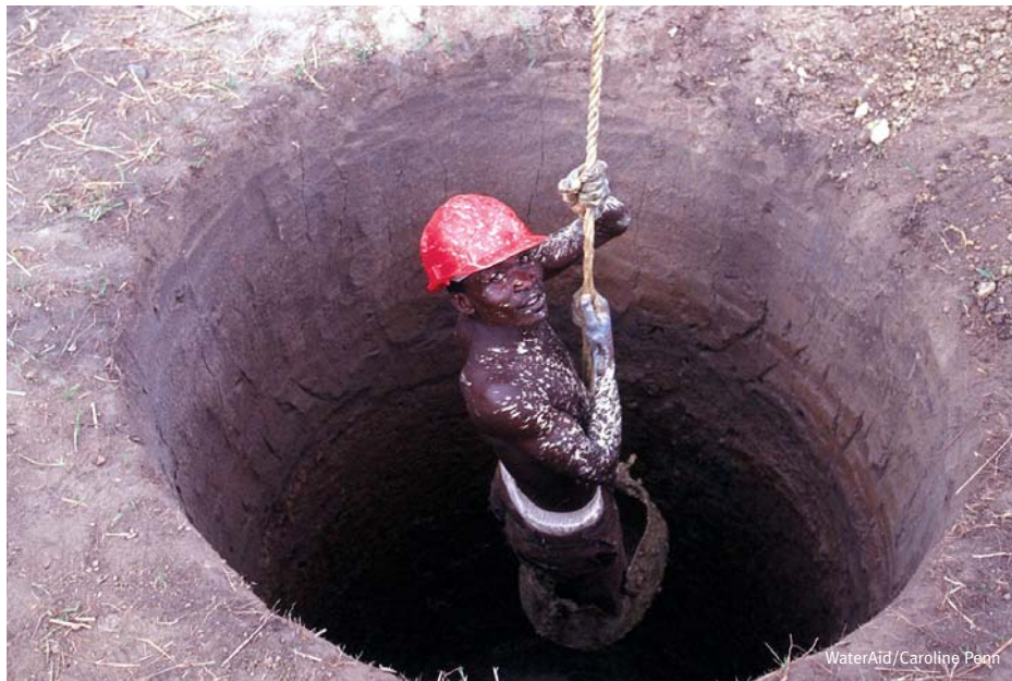
Construction of a 21 feet deep hand-dug well in Uganda.
