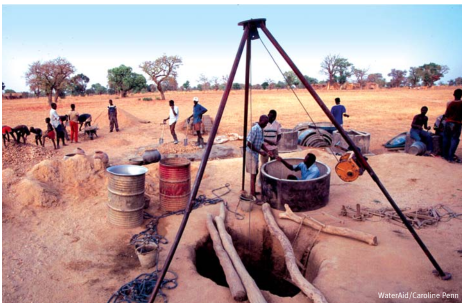
Construction of a hand-dug well in Ghana.
