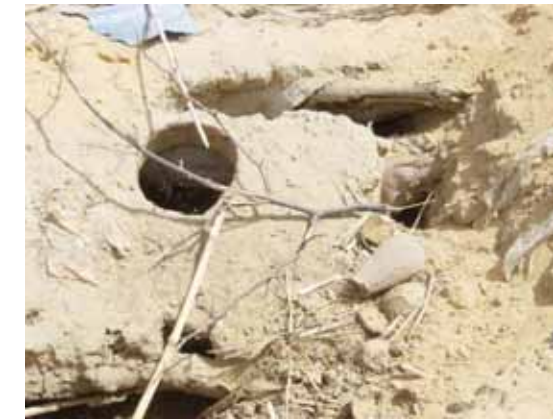
Partners and program engineers inspect a community latrine that collapsed in Benue State after a failure in the pit below (left), a collapsed pit in Jigawa State (right).
