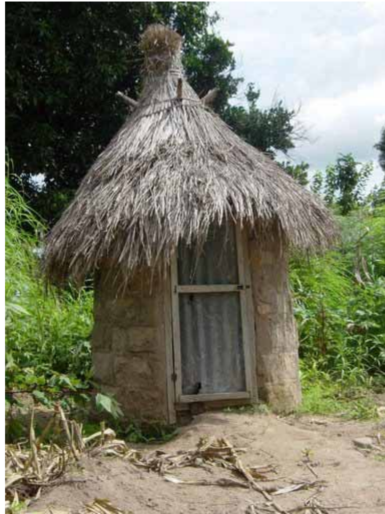
A typical pit latrine in Benue State, Nigeria
