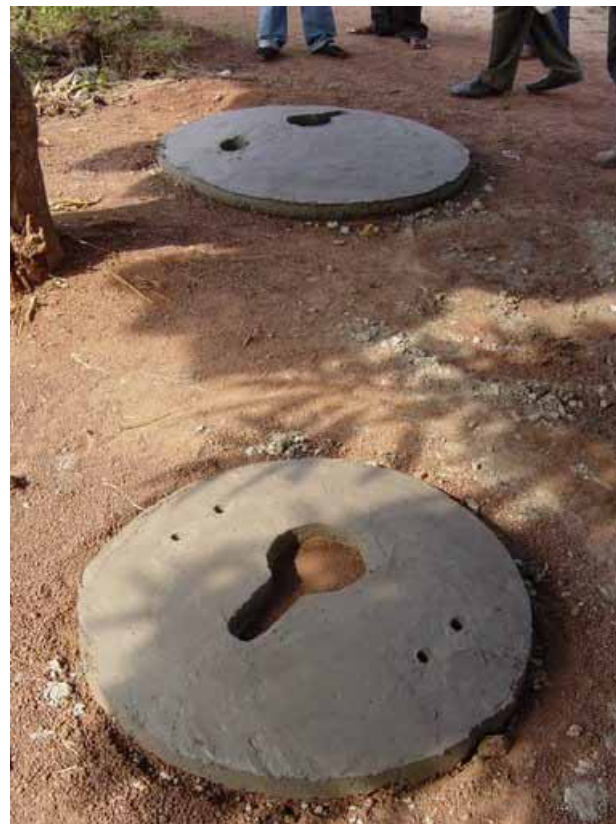
A lightweight dome slab cast in Oju LGA. Hole pairs will be used for rope handles.
