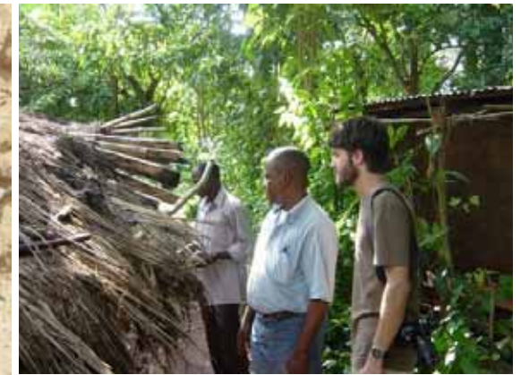
Partners and program engineers inspect a community latrine that collapsed in Benue State after a failure in the pit below (left), a collapsed pit in Jigawa State (right).
