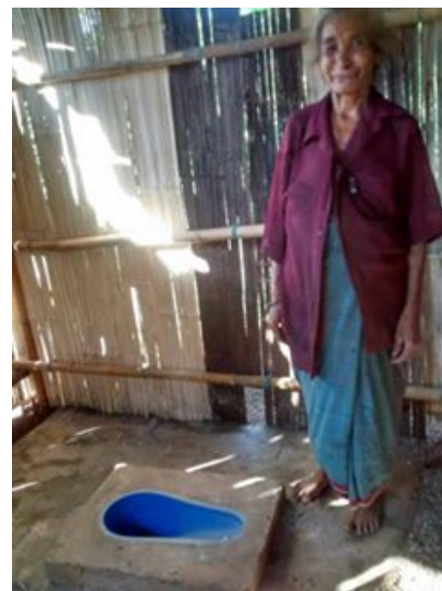
Sato Pan installation in one household, 90% of the pans from a sample of 33 follow-up households had been installed by May 2017.
