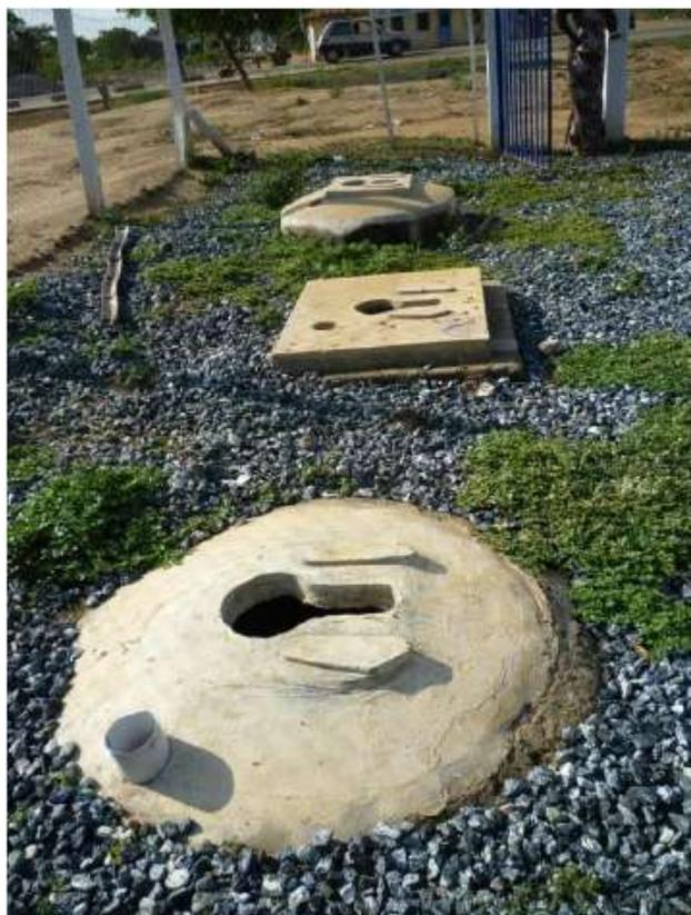
Figure 2: Sanplat models on display in the WaterAid supported sani-mart
