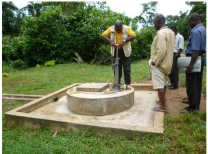
Figure 1: Protected hand-dug well in Gambia village fitted with a Nira handpump
