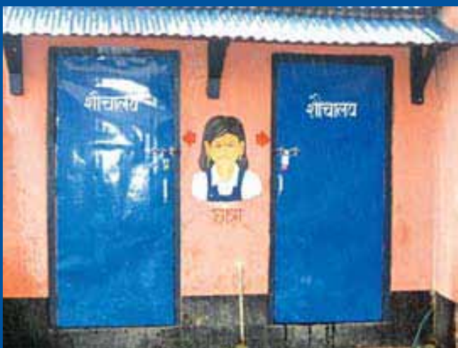
FIGURE 7. Female toilets in Bhimnagar School
