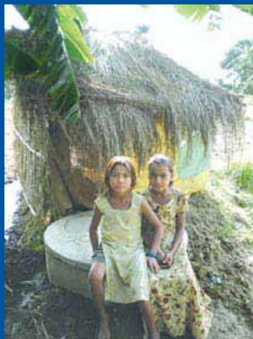
FIGURE 10. Newly completed latrine
