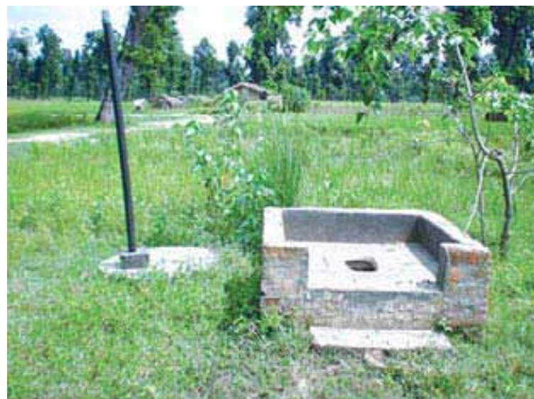
Figure 15. First-class latrine up to pan level, but not in use.
