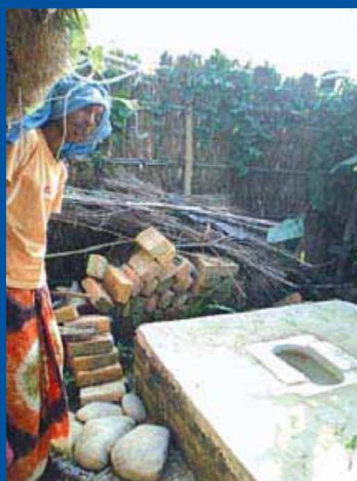
FIGURE 11. Ongoing latrines construction
