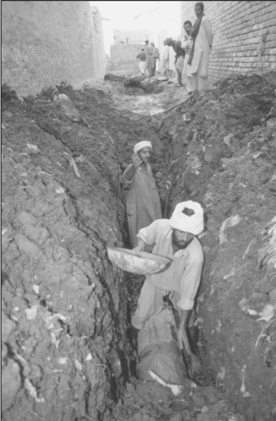
*Men dig a trench and lay pipes through compacted sewage, earth and rubbish in Hassanpura, Faisalabad.*
