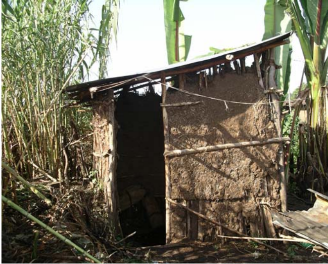
Traditional Pit Latrine visited during the study
