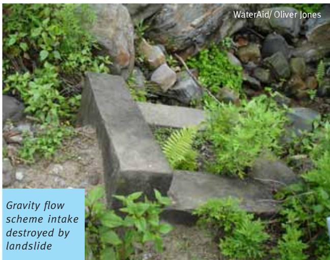
Gravity flow scheme intake destroyed by landslide
