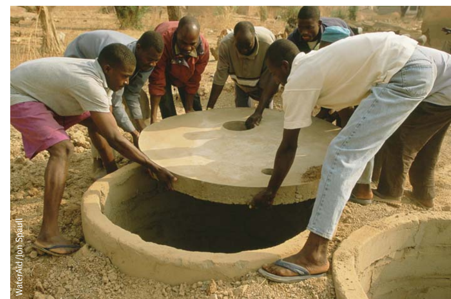
Partner staff and community members work together to construct latrines.
