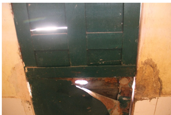
Figure 3-G. Example of broken door with peep holes.
