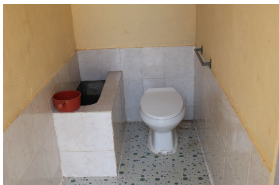
Figure 3-C. Example of grab bar on one side only inside school toilet.
