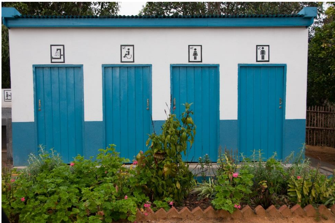
Accessible toilets in Madagascar, August 2017.
