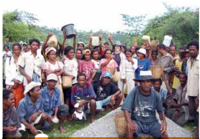
Billimau community collecting sand for their water supply construction; Bobonaro district, Timor-Leste. Photo: Claire Rowland, IDSS.
