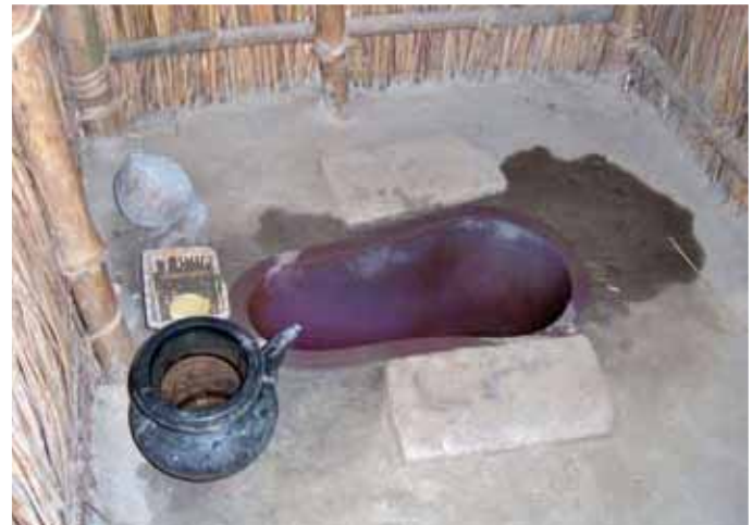
Low cost pour flush latrine, Rajshahi, Bangladesh Photo: WaterAid Australia
