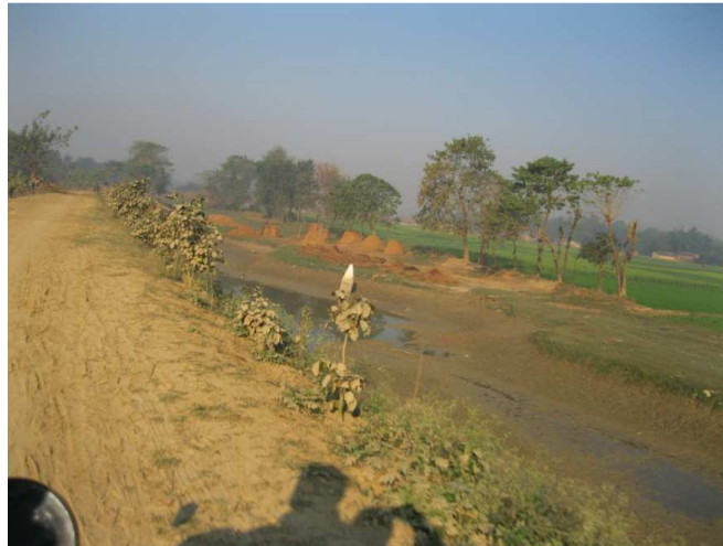
Photo: Inundation areas in Rautahat District (Banjaraha VDC)-Junge Pillar seen in subsided land. The embankment made by India causes inundation in Nepal region. The embankment has been constructed across E-W direction , that is, against flood water flowing in Lalbakaiya River (N-S direction) in monsoon season. The region is flood-prone due to the floods in Lalbakaiya River.
