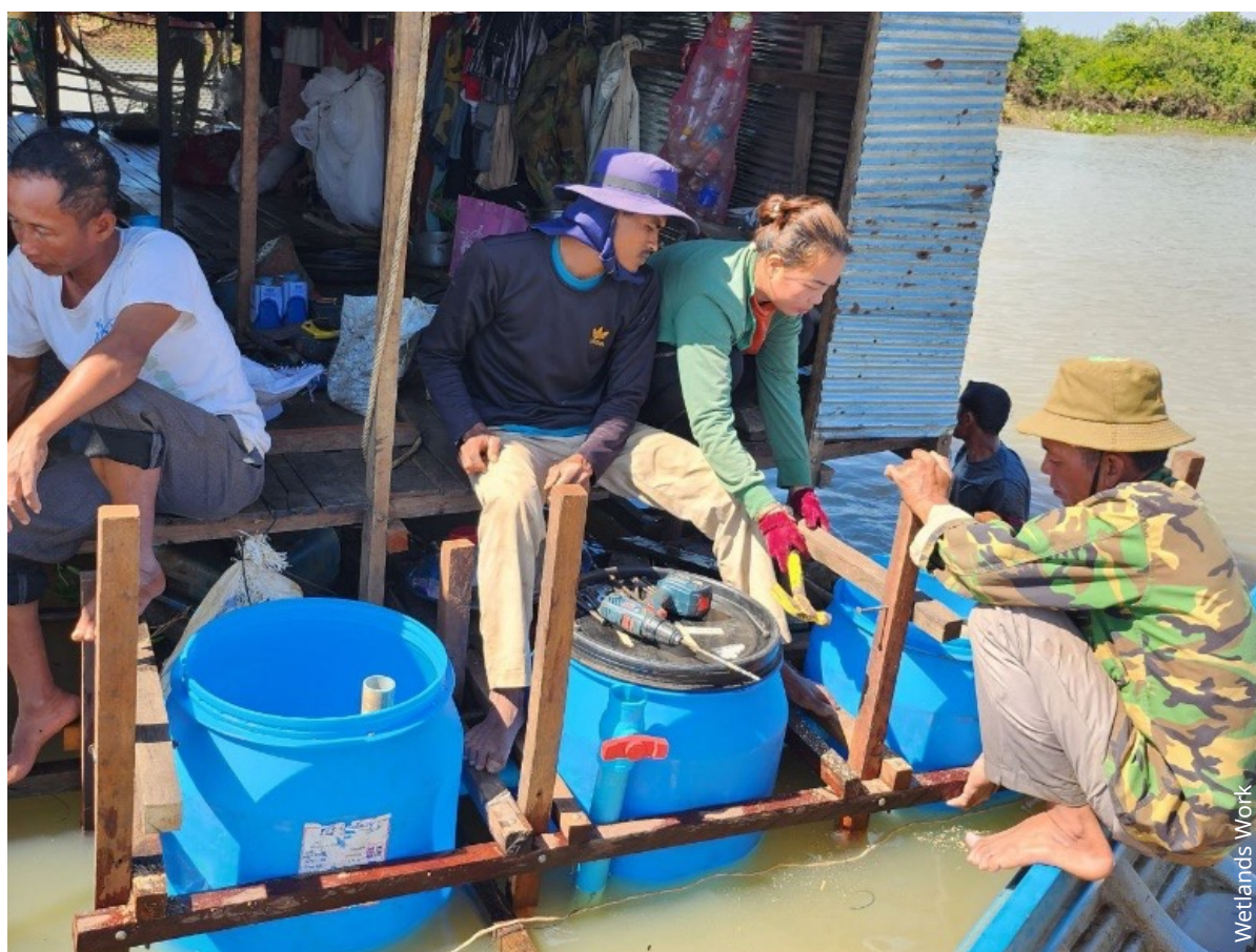
Figure 28: HandyPod installation, Wetlands Work!
