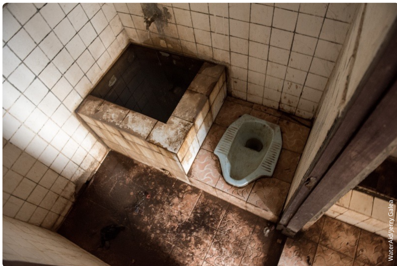
Figure 9 - Low ratios of toilets to students in many schools result in poor cleanliness and rapid failure of existing toilets.
