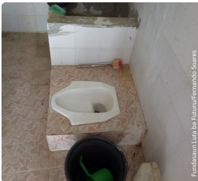
Figure 7- Many of the smaller health care facilities, such as the Liurai health post, do not meet JMP basic sanitation because they require separate toilets for staff, sex-separated toilets for patients, or accessible toilets.
