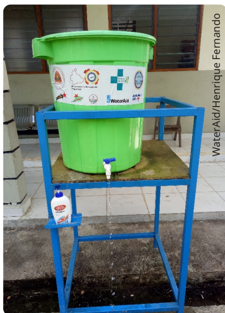
Figure 9- Bucket-tap style handwashing facilities such as this one at Dotik Health Post have proliferated during COVID-19 but have relatively life-spans before they need to be replaced, which adds significant rehabilitation costs over time.
