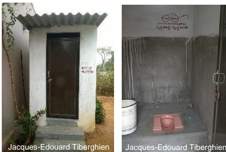
Completed toilet built with Government subsidies.
