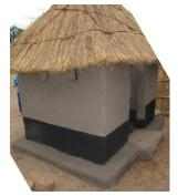
Rammed earth structure with thatched roof
