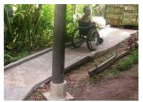
Low-gradient concrete ramp with raised sides for safety
