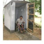
Level concrete threshold with raised cement mound to reduce flooding. Mound is rounded for wheelchair access.  Reduces water inflow without preventing wheelchair access  Won't stop serious flooding! Medium
