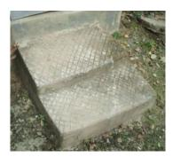
Low concrete steps • with cross-hatching to reduce the risk of slipping
