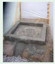
Sanitary pad washing slab inside screened unit
