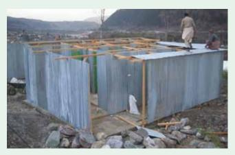
Warm bathing unit under construction – laundry area seen to the front and right of the picture
