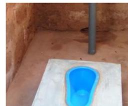
A traditional Ventilated Pit Latrine (VIP) converted to a Water Easy Toilet by installing only the offset.
