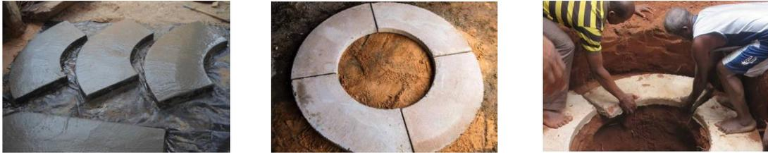
A four-piece crescent shaped concrete placed on the neck of the pit to prevent caving in. They can also be called the parapet.
