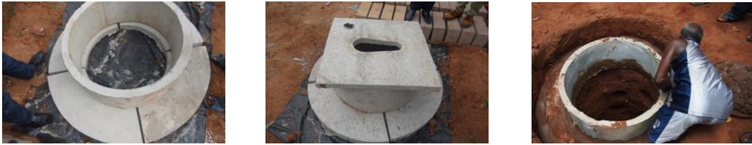
This is a concrete place at the neck of the pit. It is a stool for the direct pit slab. The pit slab is placed on the ring before filling the neck of the pit.
