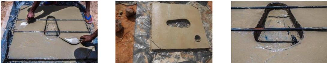
This is the final concrete component placed on the ring. It has the cone-cut provision for the SaTo Pan to fit in.
