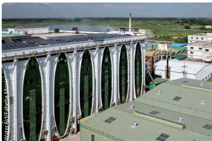
● The rainwater harvesting system at Fakir Fashion has helped reduce the factory's dependency on groundwater. Narayanganj, Bangladesh. October 2021.
