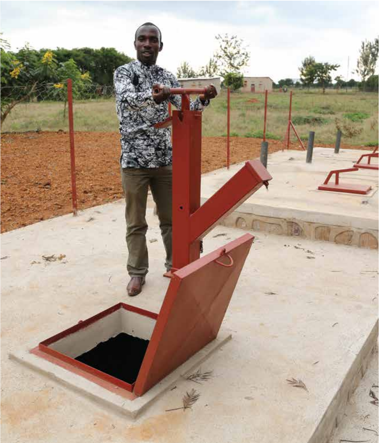
Edison, head of the Nzangwa Health Centre, shows the newly built medical waste disposal site, which also has a bottle crusher
