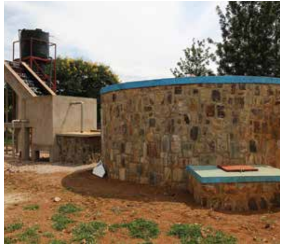
One of the reservoirs WaterAid Rwanda built has an aeration and filtering facility built into it.
