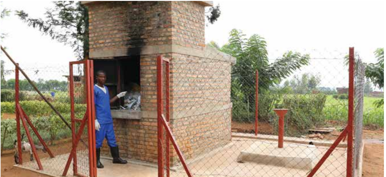
Eric 23, a full-time janitor at Nzangwa Health Centre shows how waste is discarded using the newly renovated burner done by WaterAid.
