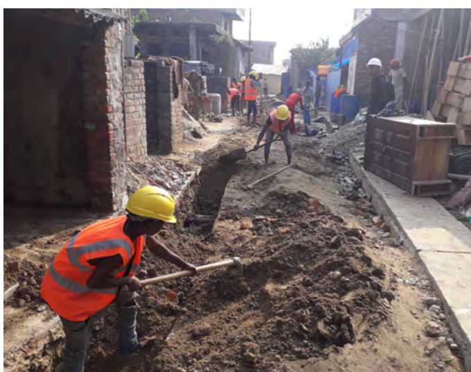
NWSC installing pipeline in Lahan municipality.
