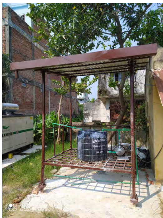
Figure 7: Temporary chlorine dosing system (photo) and proposed solution (drawing).
