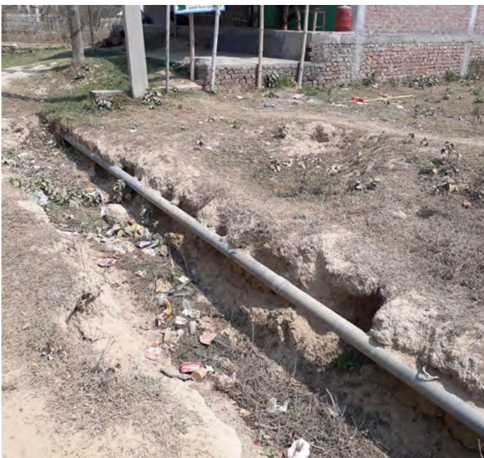
Damage to pipes due to the shallow depth.
