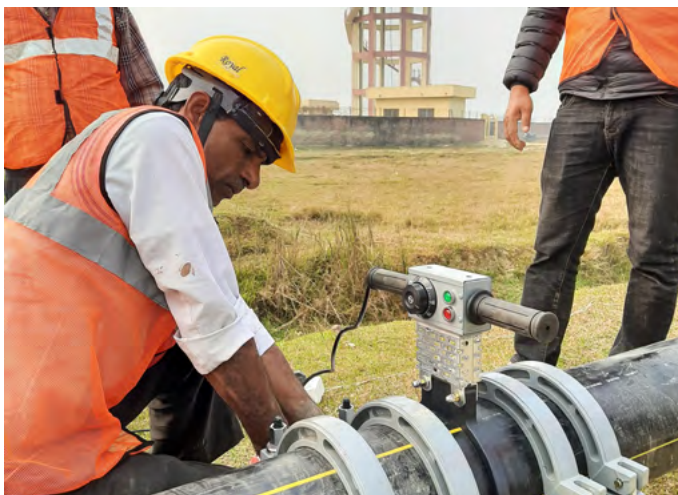
Figure 9: Welding high density polyethylene (HDPE) pipe.
