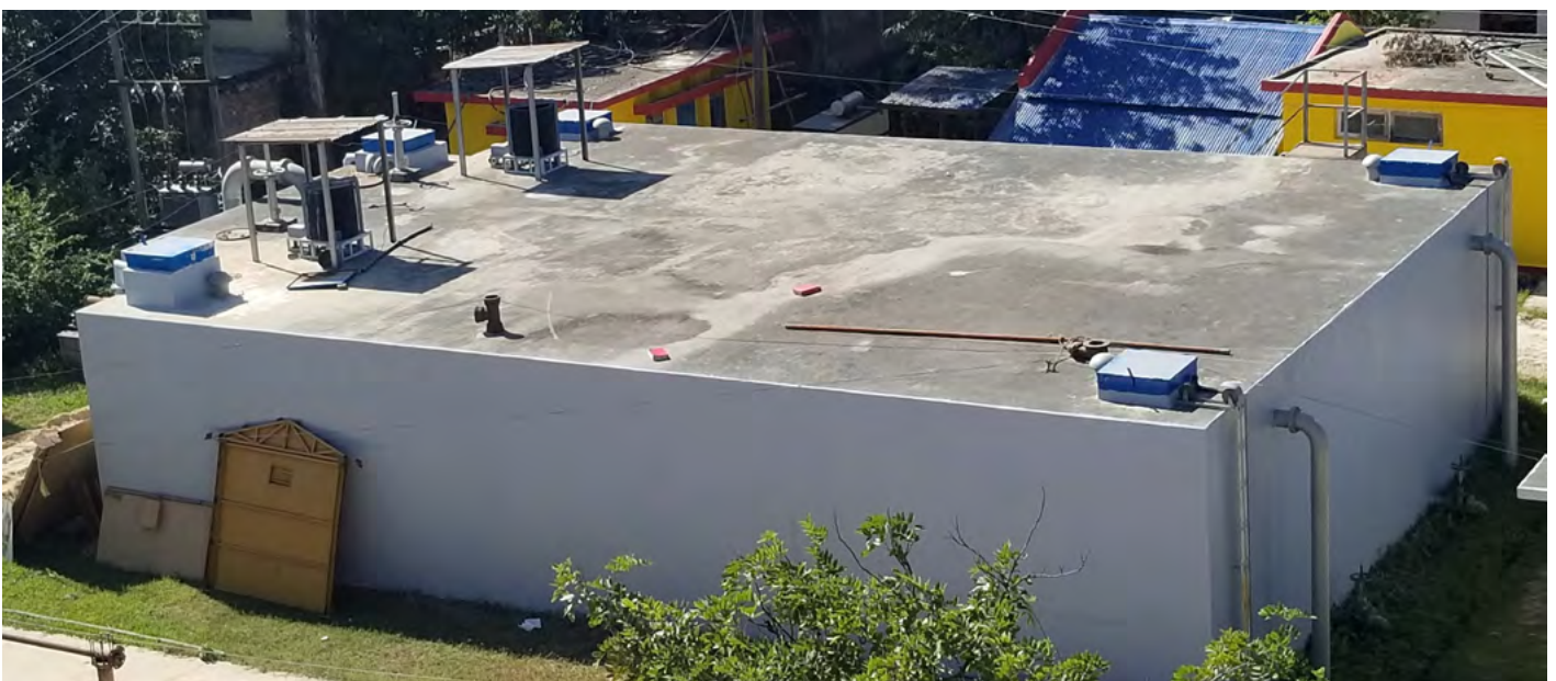
Rehabilitated sedimentation tank with the new hatch covers.
