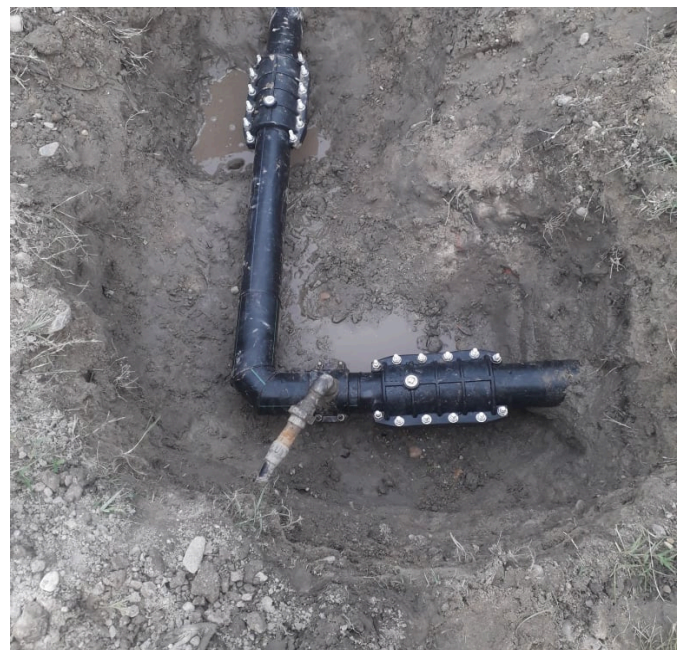
Leakage repair and household connection.
