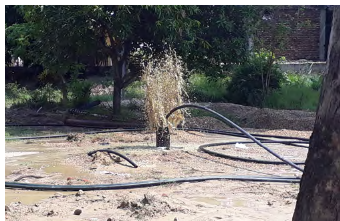
Using an air compressor to complete the development of BH7.
