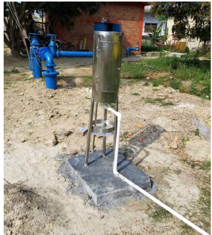
Borehole sampling tap installed in NWSC Lahan.
