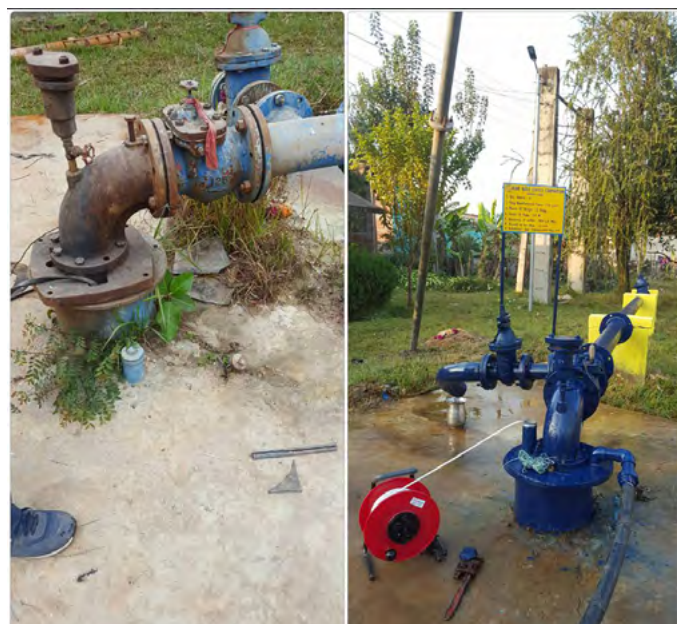
Before and after replacing borehole head plates.
