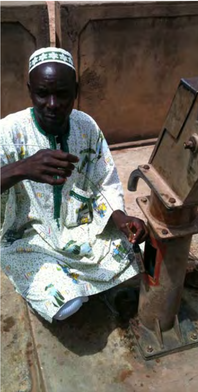
Figure A7 Installation of a water level logger inside a borehole in Burkina Faso. (Credit: Vincent Casey/WaterAid).
