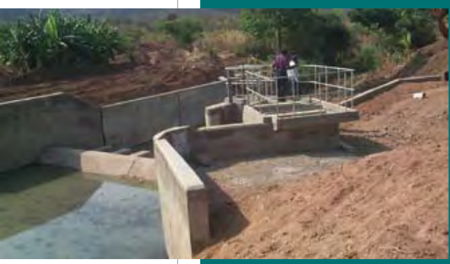
Figure 7.2 Example of an improved modernised irrigation intake in Usangu, Tanzania (Credit: Bruce Lankford, UEA).
