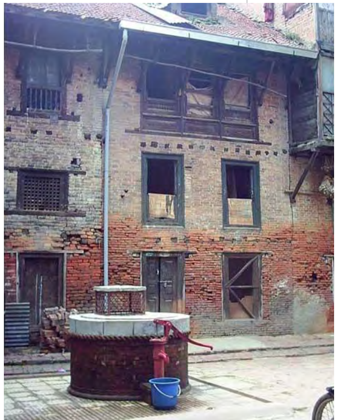
Figure 6.3 Example of a recharge well and connecting rainwater harvesting system in Patan City (Credit: Kabir Das Rajbhandari, WaterAid in Nepal).
