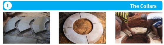
A four-piece crescent shaped concrete placed on the neck of the pit to prevent caving in. They can also be called the parapet.
