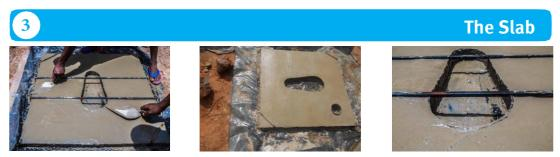
This is the final concrete component placed on the ring. It has the cone-cut provision for the SaTo Pan to fit in.
