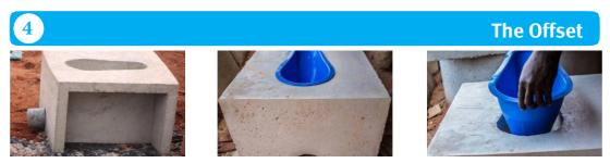
This is the box-like concrete component and can be installed in the home. It is connected to the pit through a PVC pipe and can be enhanced or modified to serve as a semi Water System. It is also fitted with the SaTo Pan.
