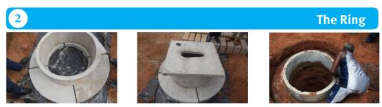
This is a concrete place at the neck of the pit. It is a stool for the direct pit slab. The pit slab is placed on the ring before filling the neck of the pit.
