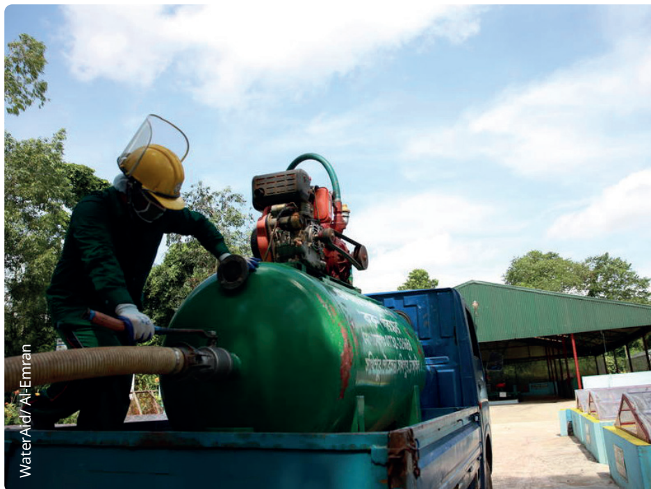
▲ Fig.5: A worker prepares to empty a Vacutag sludge pump in Sakhipur
