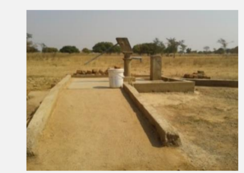
An accessible waterpoint in Zambia. It has a ramp, with raised sides to ensure wheelchair users don't fall off and which people with visual impairments can use as a guide. It also has a water bucket resting stand.
