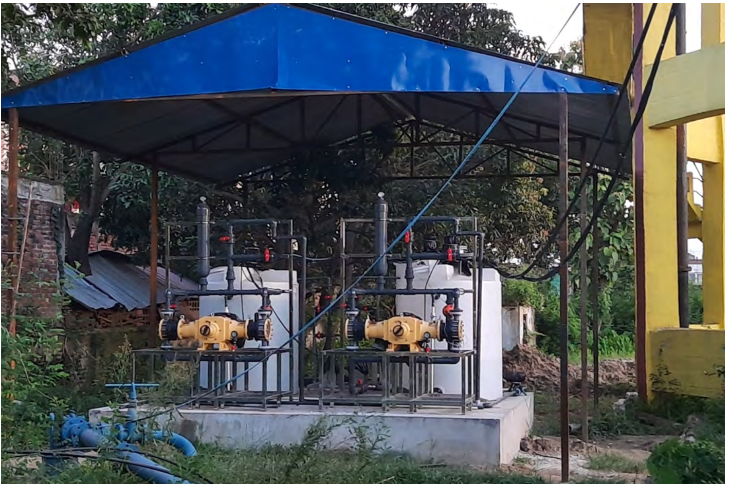
Chlorine dosing system installed in the NWSC compound
