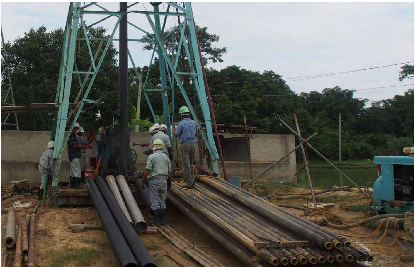
Lowering casing for the new borehole recently drilled in Ward 9
